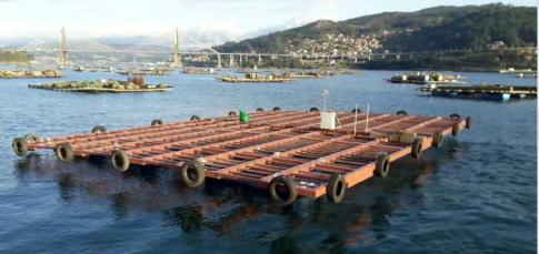
Since 2018 and under the H2020 project ReSHEALience-760824 (www.uhdc.eu) an intense work is being developed to estimate the real durability of structures in XS and XA aggressive environments. A TRL7 540 m<sup>2</sup> UHC raft will be floated in Valencia with continuous monitoring including a continuous measurement of the strain in the beams. Some of them are designed to suffer micro-cracking under service to evaluate the level of self-healing reached with different concrete mixtures.
